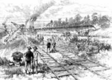
Excavation of Panama Canal near Tabemilla
